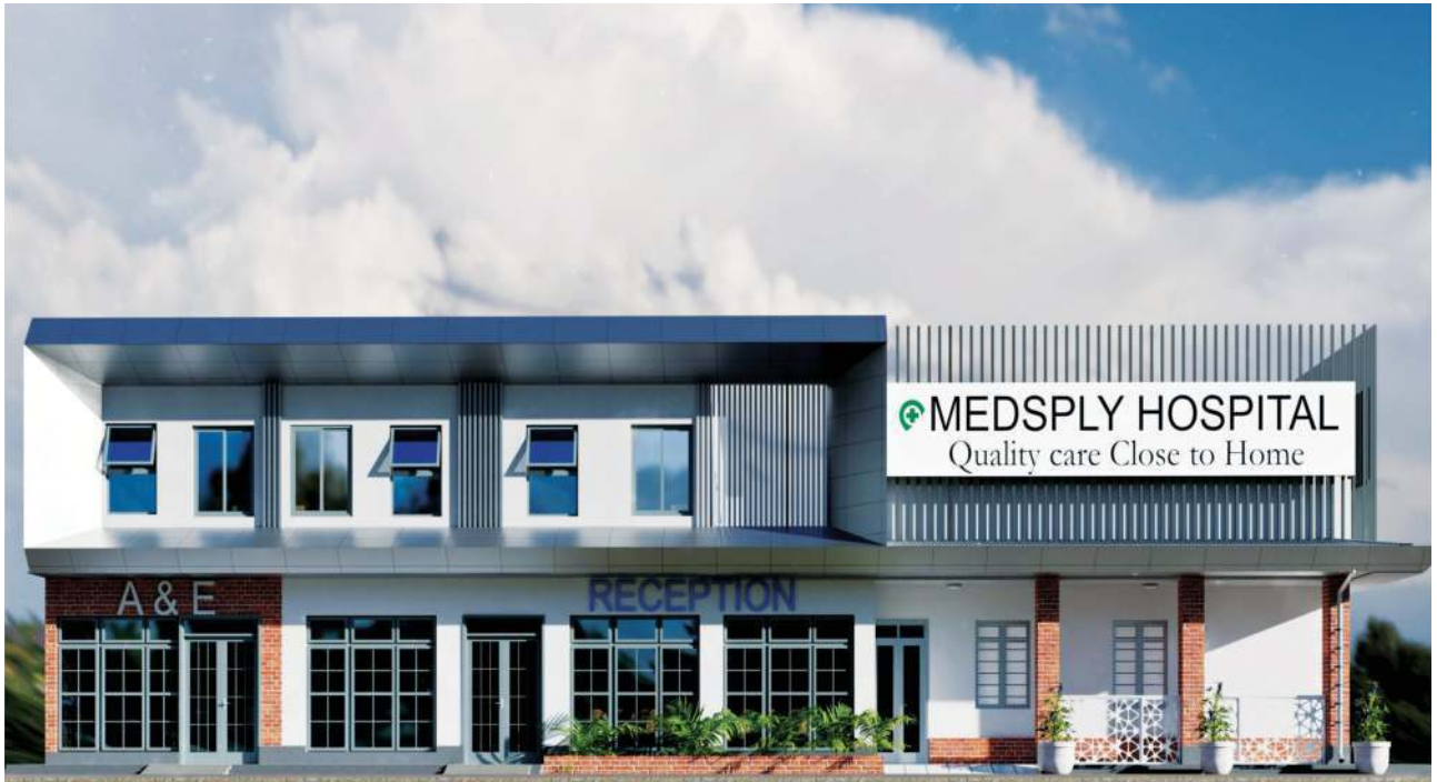
Design and Build of Medsply Hospital, Mumias
