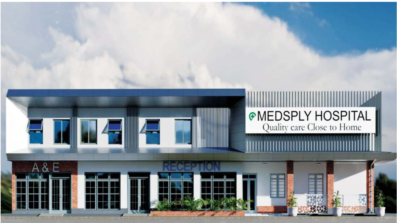
Design and Build of Medsply Hospital, Mumias
