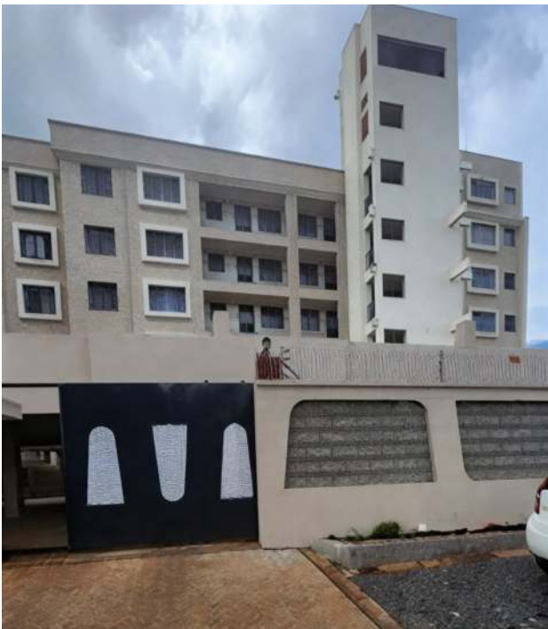
5 storey apartment in Ruaka
